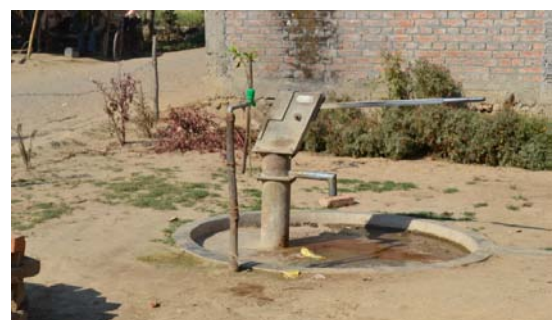
Deep bore Hand pump & tap connection in Arsenic affected village of Gangapur, District: Ballia
